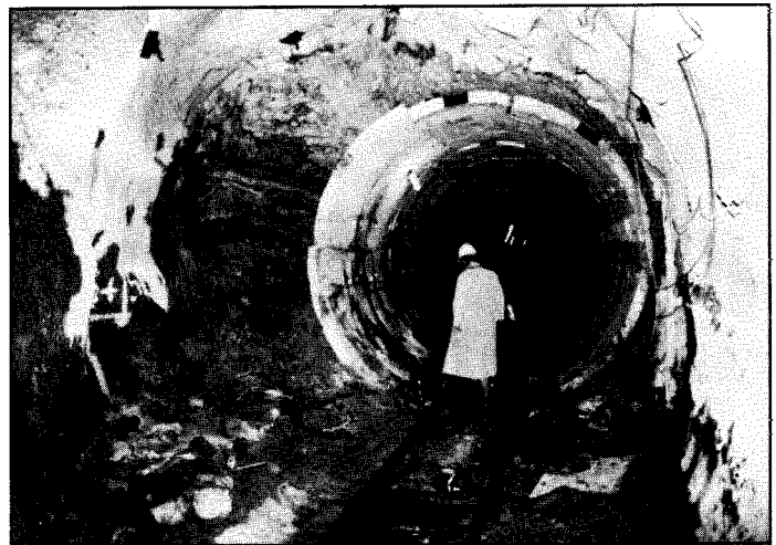
Fig 8 Illustration of overbreak (TDLR)
