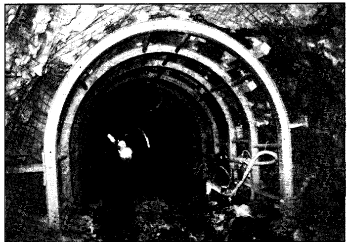
Fig 9 Illustration of overbreak (LD&T)
