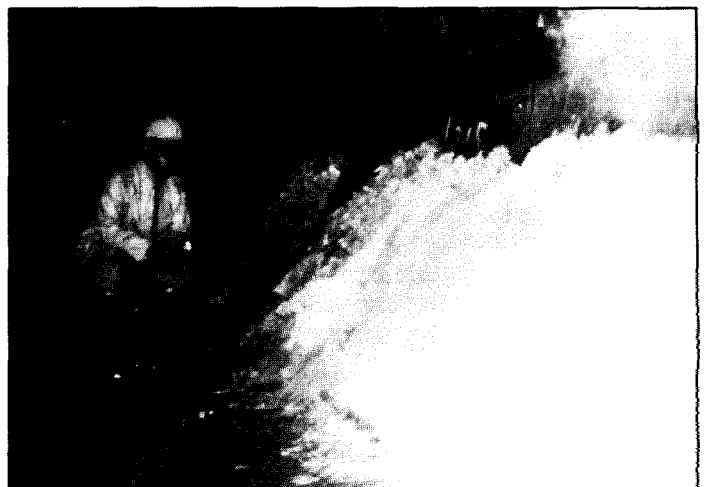
Fig 6 Stability behind work area (flowing sand)
