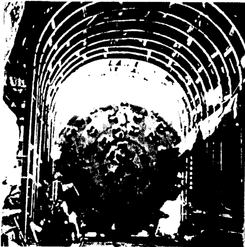
FIGURE 1: ROGERS PASS RR TUNNEL
