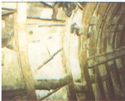
Support of shear zone, Hunter Tunnel.
