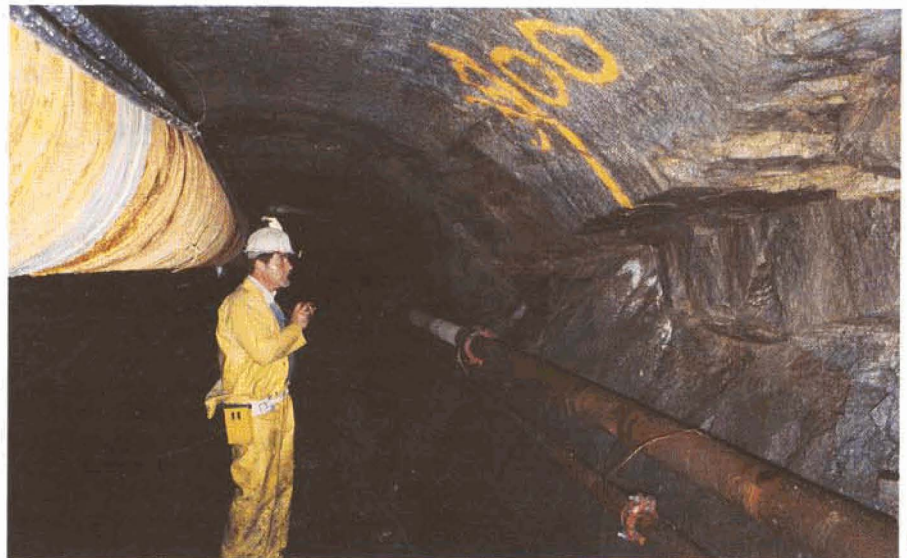
Shear zone and rock block fallout in TBM bored tunnel, responsible for delays illustrated in Figures 3 and 7.
