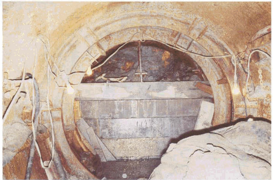
Heading of pipe jacking showing silt on the project illustrated in Figure 1.
