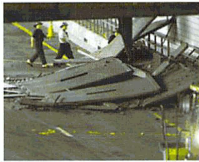
Exhibit 4: Support Elements and False Ceiling Collapse
