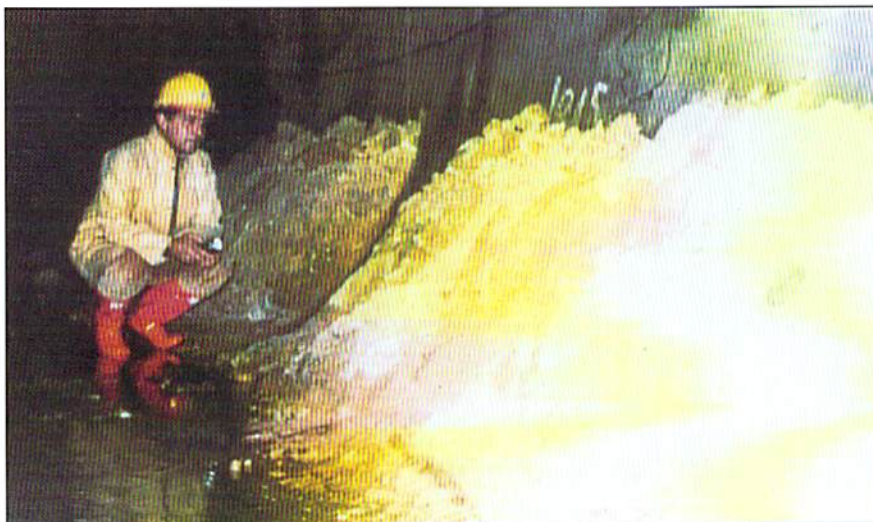
Weak sand washed through precast segment grout holes (Project 2).
